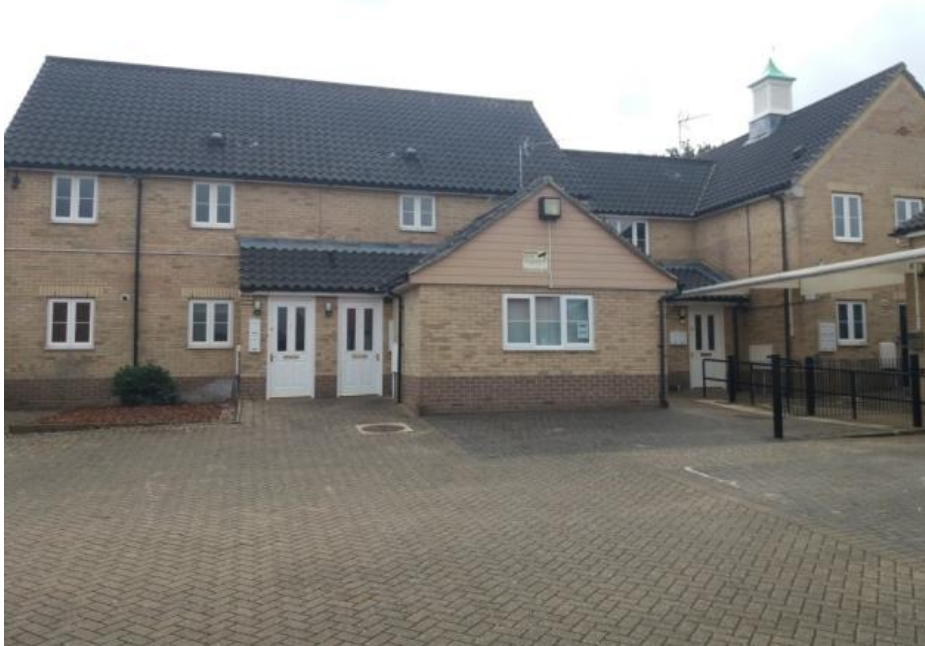
The refurbished Foyer in Stowmarket will be help reduce the dependency on B&Bs Picture: MID SUFFOLK DISTRICT COUNCIL
